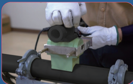
새들 융착 SADDLE WELDING
